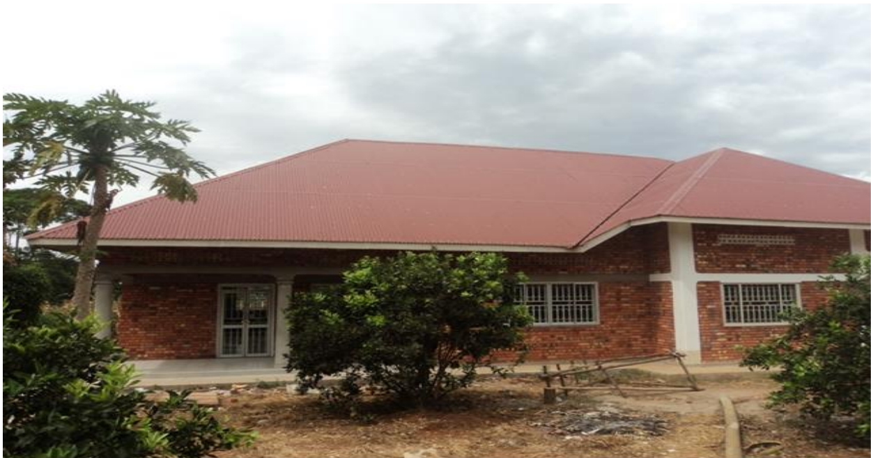
Photo 5: showing the newly constructed MDMS Store block standing between remnants of the Orchard before the packing area was created.
